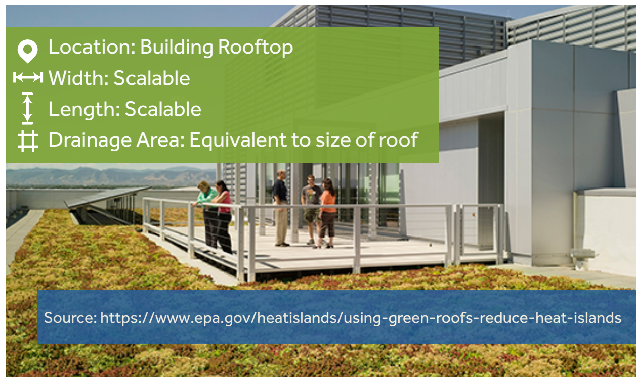
Figure 9: Green roof in urban setting
