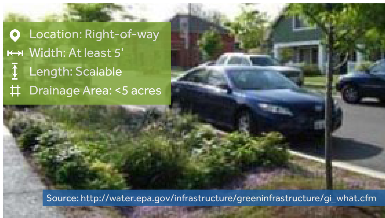
Figure 5: Bioswale in a suburban setting
