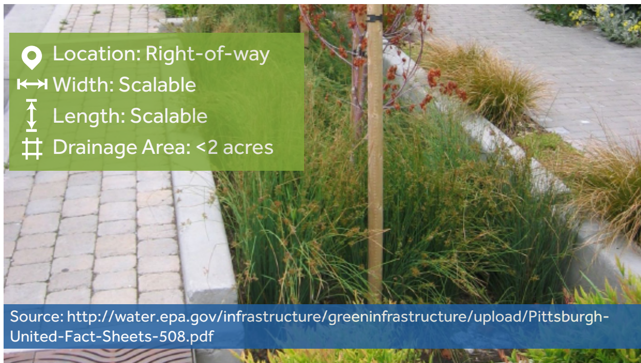
Figure 7: Stormwater planter in a suburban setting
