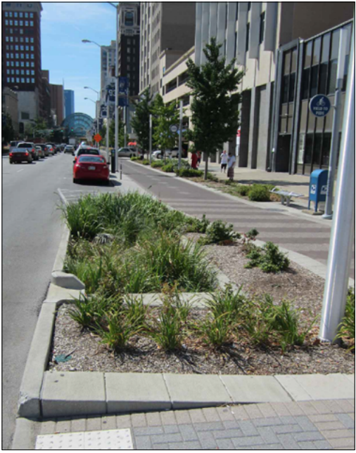
STORMWATER PLANTER INSTALLATION 5, 6
